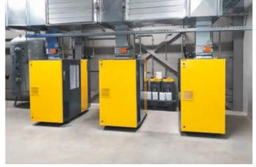
KAESER ASD 40 T rotary screw compressors with heat recovery.
