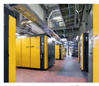
A total of four rotary screw compressors with IE4 drive motors and the energy-saving SIGMA PROFILE operate in the compressed air system.
