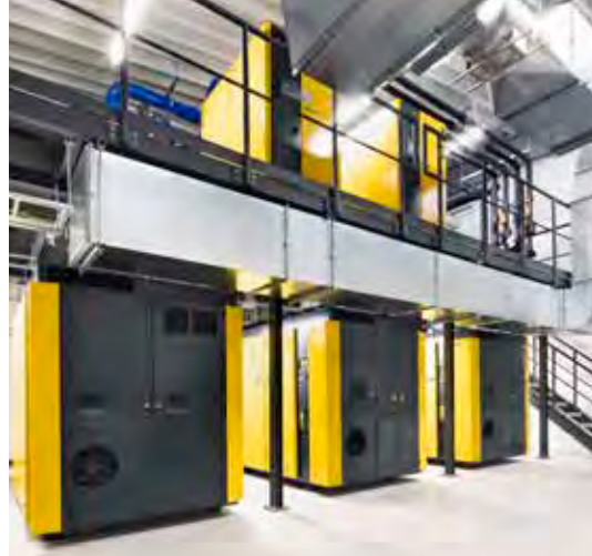
Image, left: Huge sheets of foil are produced inside these towering extruders. Image, right: The new compressed air station is arranged on two levels to save space.
